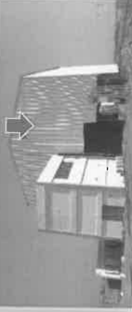
GI Sheets , dust collector provided around all wagon tippler area to control dust emission
